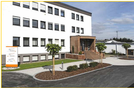
Main building in Langenfeld
